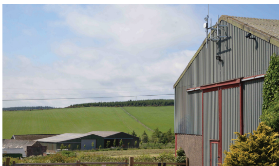
A SmartRural mast in situ on farm.
